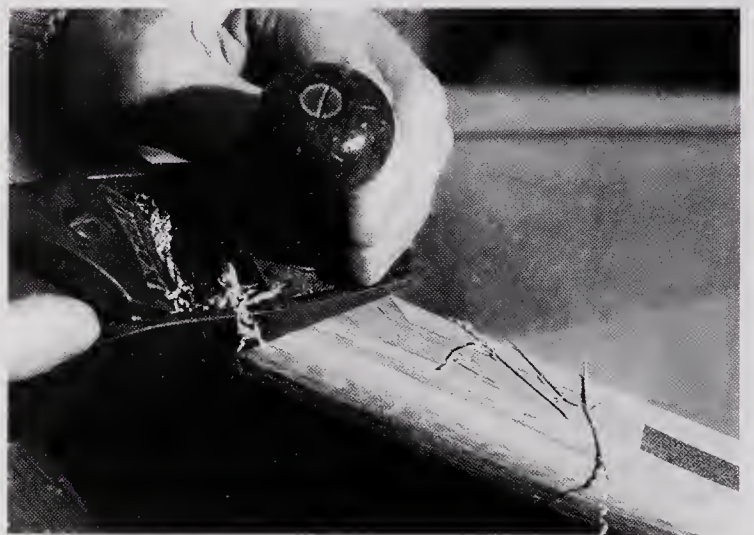
The top of the breasthook is rounded off neatly and is faired into the top of the gunwale.
