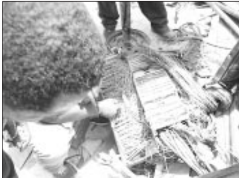
Technicians working on the cables that will be rejoined today.
